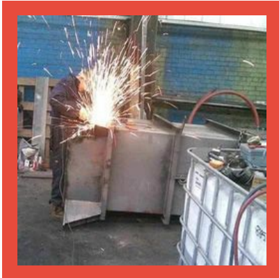
Stainless Steel Fabrication Job Works
