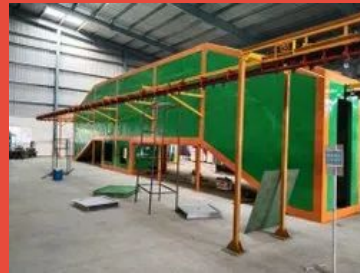
Powder Coating Plant
